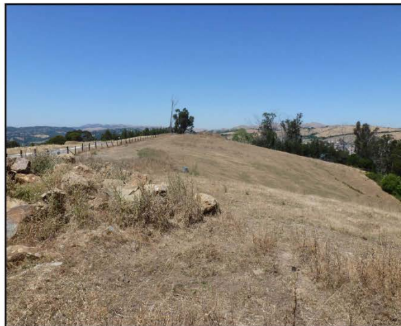
Figure 5b. Looking north
